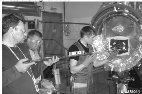
Fig. 6.5.4 Installing the new liner on the 3.5 T multipole wiggler on the Diamond Light Source storage ring (England).
