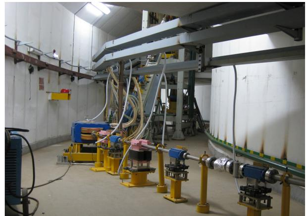
Fig. 5.3.4. Descent of beams in the tunnels for the beam transport lines of the injection complex.
