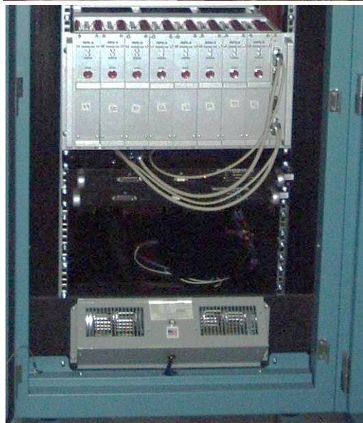
Fig.5.13.14. Power supplies for the quadrupole magnets (above). Power supplies for the corrector and sextupole magnets (below).
