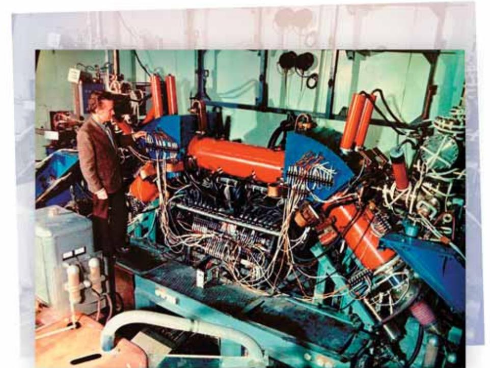
1976. The heart of the HAP-M system is the EPOKHA setup based on the electron cooling method and one of its founders, V. I. Kudelainen
